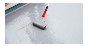
A minimum of three (3) coating applications of **FORTRESS** must be applied on the surface. Stir well before using. Curing time per coating application is 2 hours.
