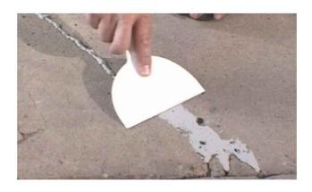
All visible cracks should be sealed properly using **GreenSeal Waterproof Elastomeric Sealant**.
