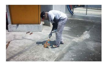
Surface must be clean, dry, stable and free from dirt, dust, oil, grease and other contaminants that will impede on the proper adhesion of the coating. New concrete structures need to be cured for at least 28 days prior to application.
